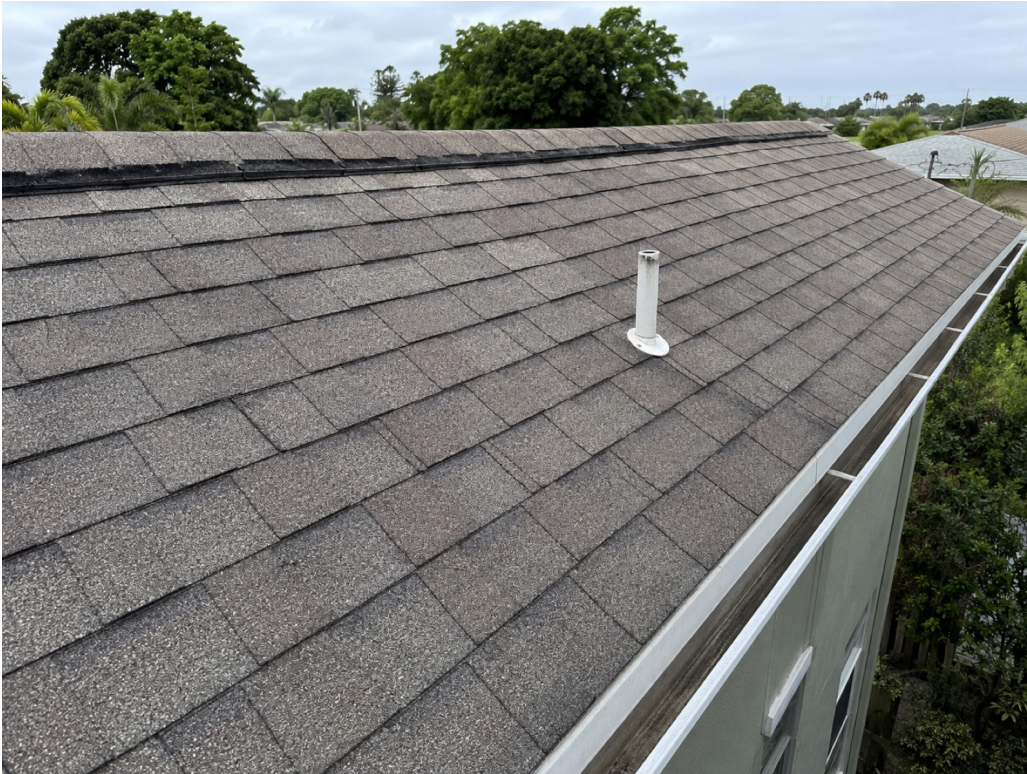
Q2 Roof Covering — photo 1
