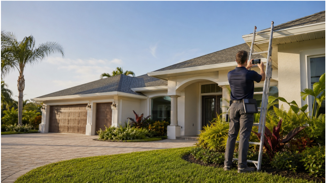
Q5 Roof Geometry — photo 1
