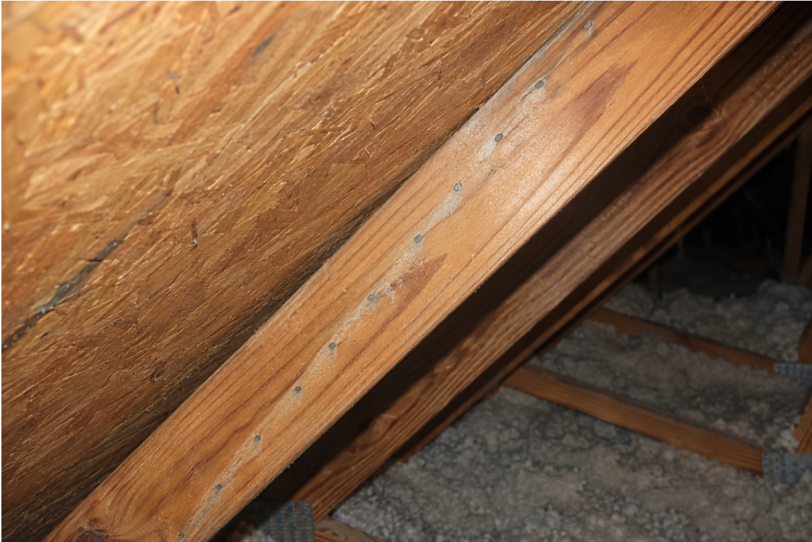
Q3 Roof Deck — photo 2
