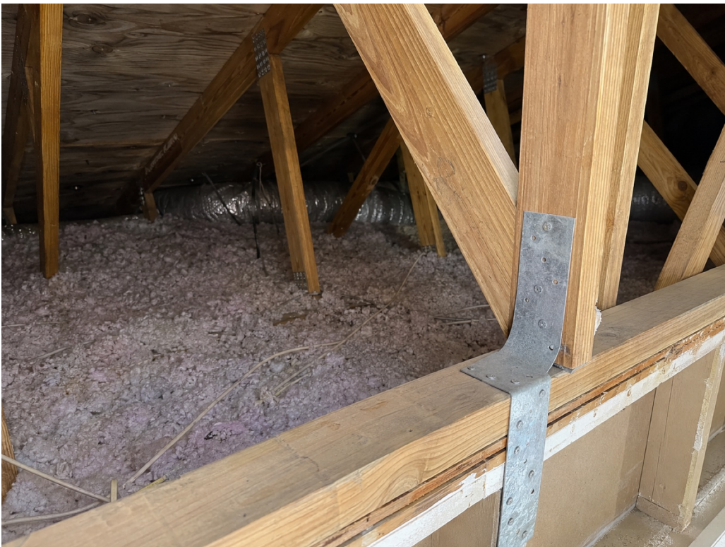
Q3 Roof Deck — photo 1
